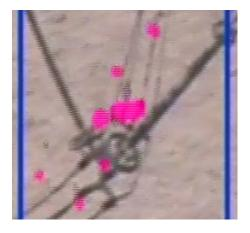
Excessive corona discharge on insulators
